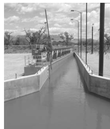
Water intake structure with fish screens.
