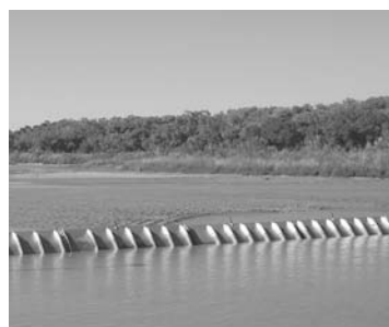
It takes about three hours for water to travel from the diversion dam (pictured on left) to the settled water ponds at the surface water treatment plant. After settling for at least a day in the ponds, it only takes two or three hours of treatment to produce the clean, finished drinking water pictured on the right.
