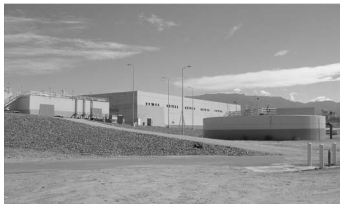
The surface water treatment plant.
