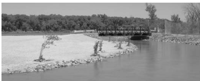
Fish passage at diversion.
